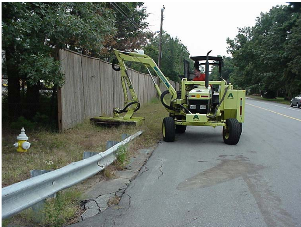
TYPICAL MOWING OPERATIONS
