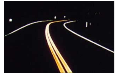
Example of highly retroreflective pavement markings at night. (Source: FHWA)
